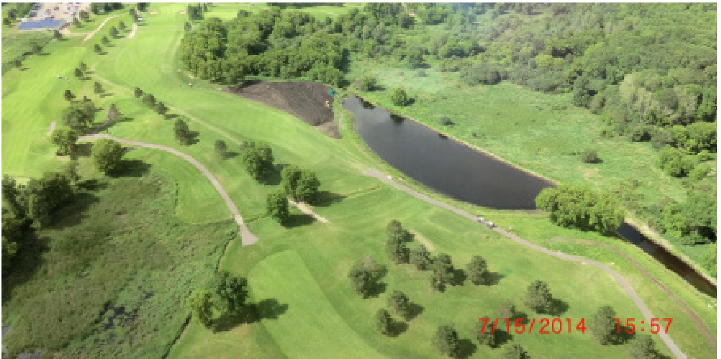
The newly created containment pond on Oneka Ridge Golf Course captures phosphorous laden water from urban and agricultural runoff.
